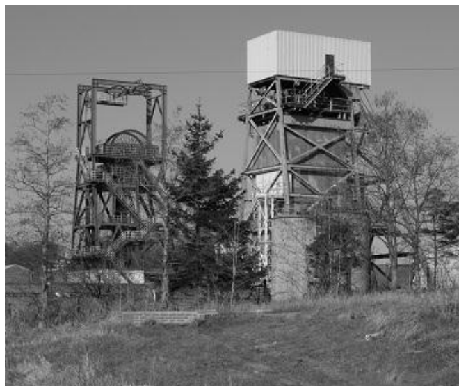
Daw Mill No 1 & 2 shafts 02/03/2013
