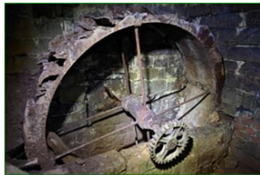
Remains of an underground iron overshot waterwheel at Tixall. (Kelvin Lake)
